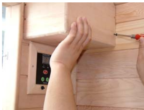
FIG-22.1 Fix the CD player back cover with screws
