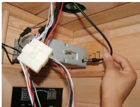
FIG-21 Link the antenna connectors
