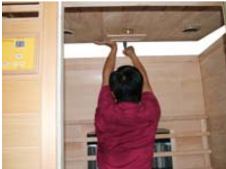
FIG-14 Setting the top board
