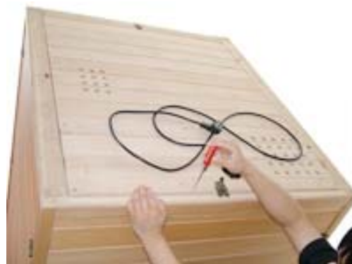
FIG-24 Fix the external board with screws
