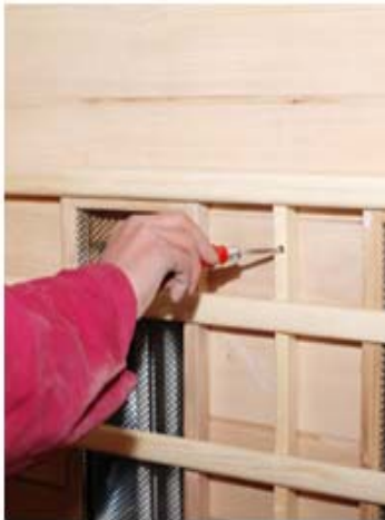
FIG-11 Assembling sitting board
